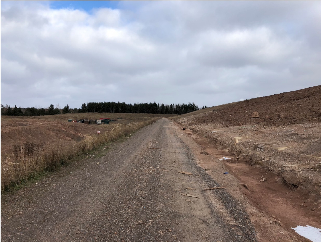
Photo 15: Location 8 – Looking North, Phase 3 LF Western Road
