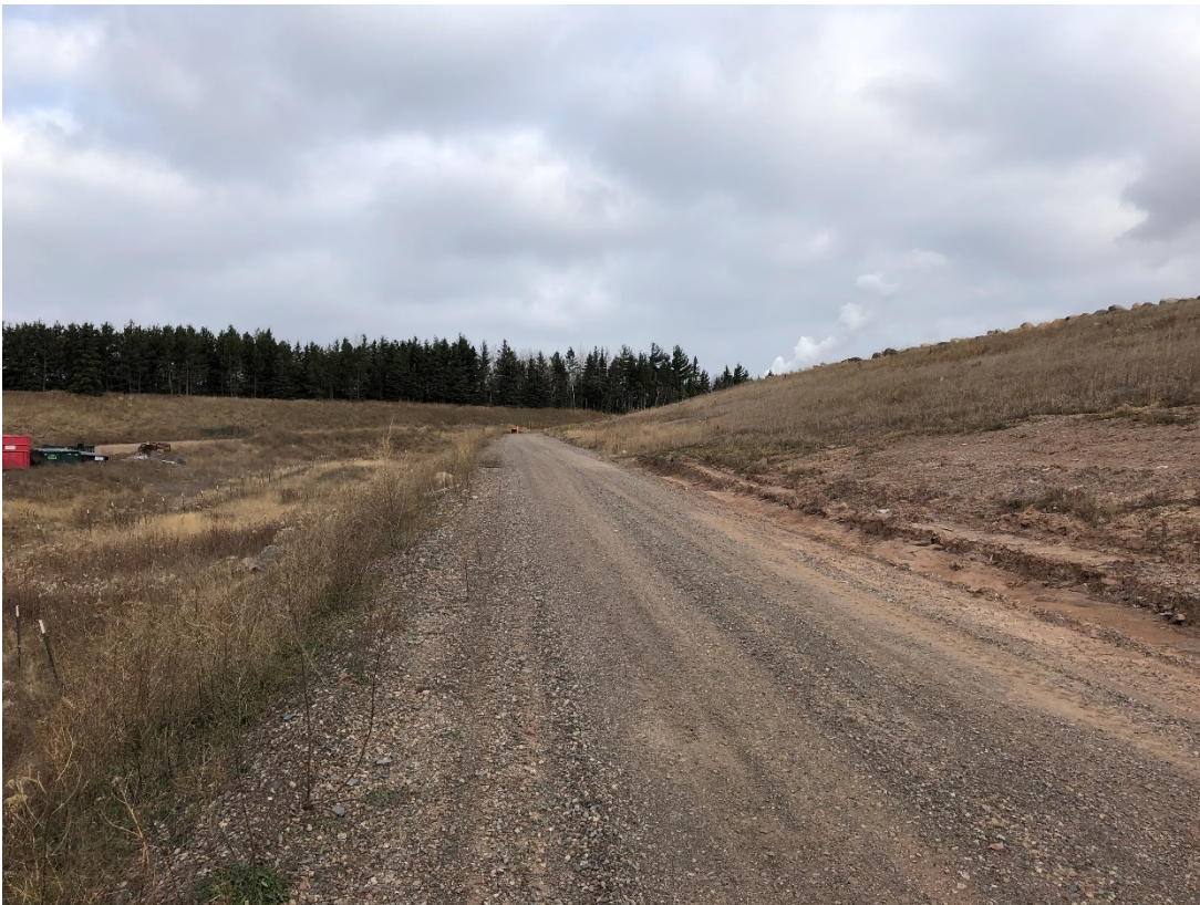
Photo 18: Location 9 – Looking North, Phase 2 Perimeter Road
