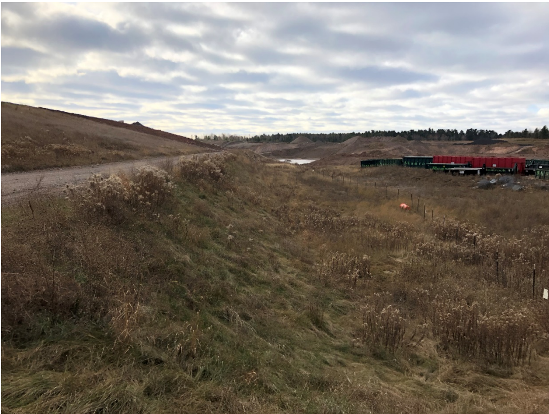
Photo 24: Location 10 – Looking South, Phase 2 Western Berm
