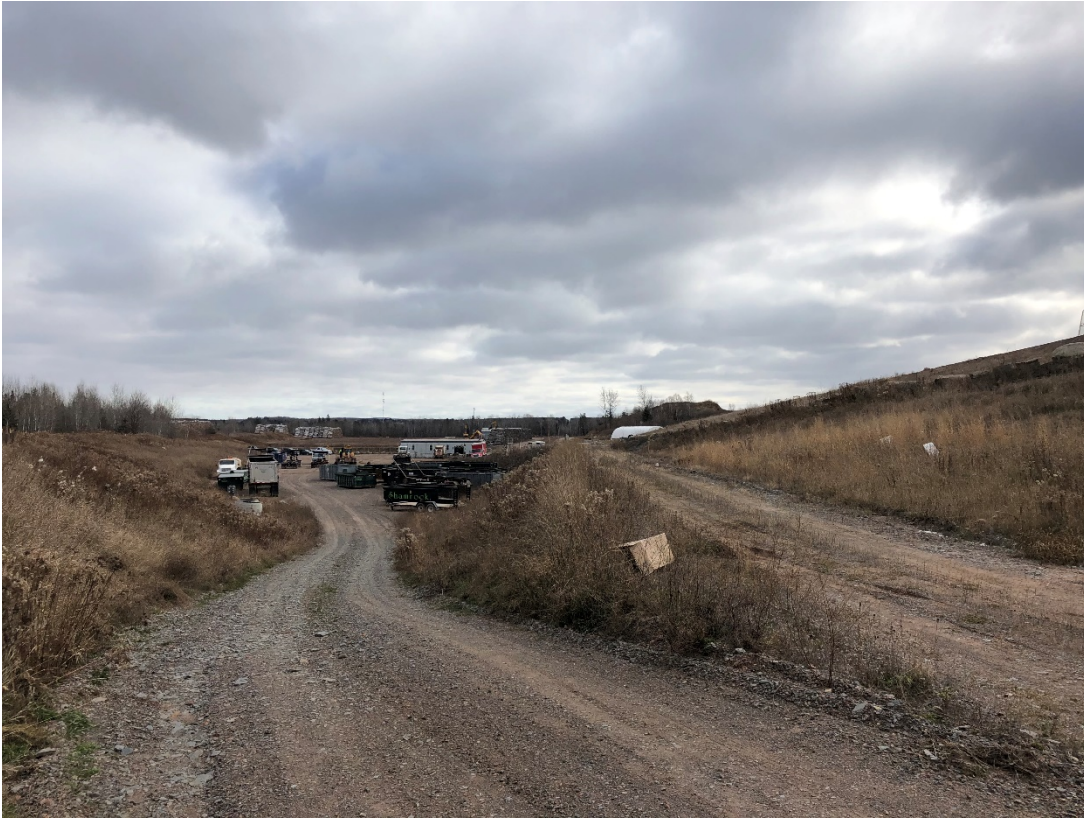
Photo 25: Location 10 – Looking East, Phase 2 Road & Berm
