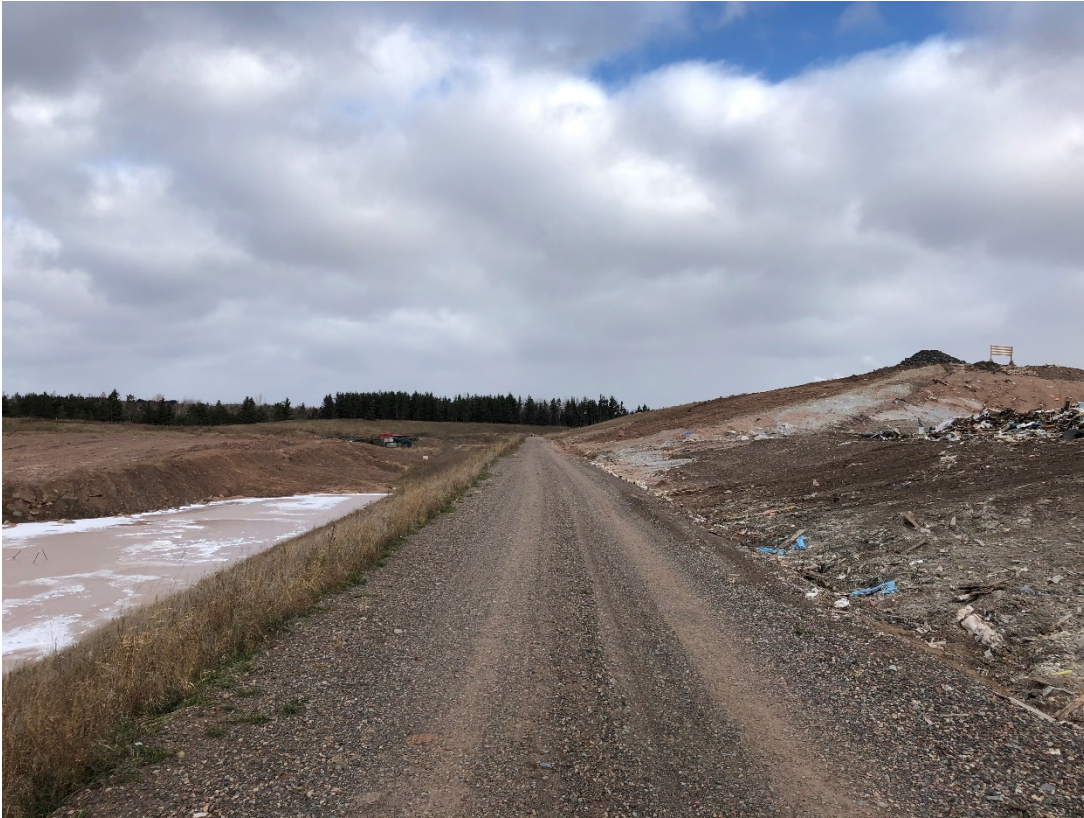
Photo 29: Location 11 – Looking North, Phase 6 Interior (Future Waste Slope)7
