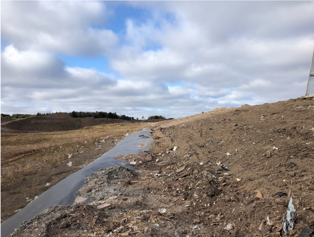
Photo 31: Location 13 – Looking West, Cell 7A Southern Rain Flap
