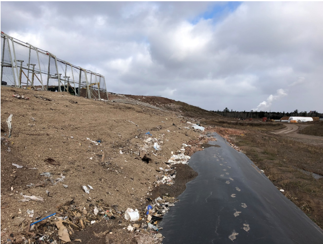
Photo 32: Location 13 – Looking North, Cell 7 Eastern Berm
