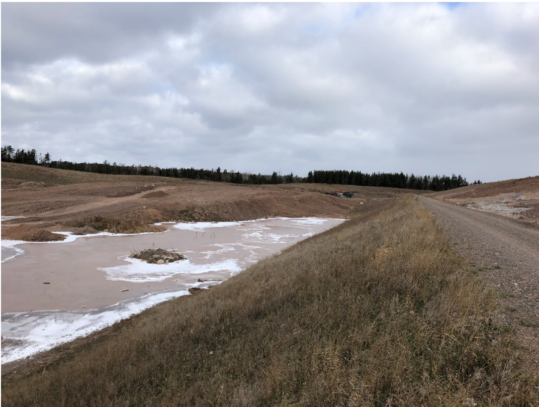
Photo 26: Location 11 – Looking North, Phase 6 Western LF Berm
