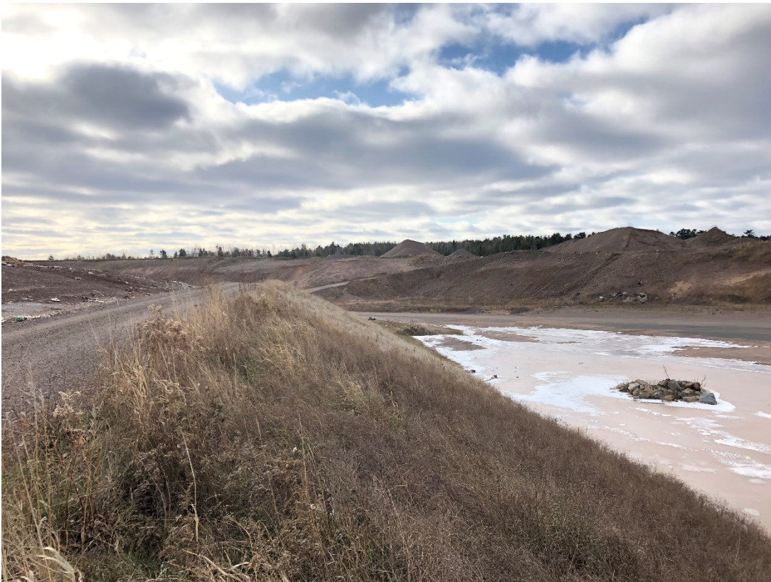
Photo 16: Location 8 – Looking South, Phase 6 Western LF Berm
