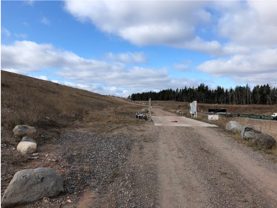
Photo 7: Location 4 – Looking West, Phase 1 Northern Berm
