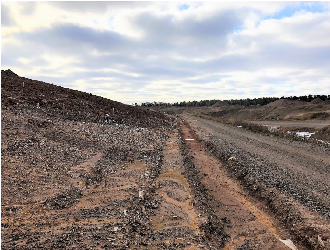
Photo 22: Location 9 – Looking South, Phase 3 Waste Slope
