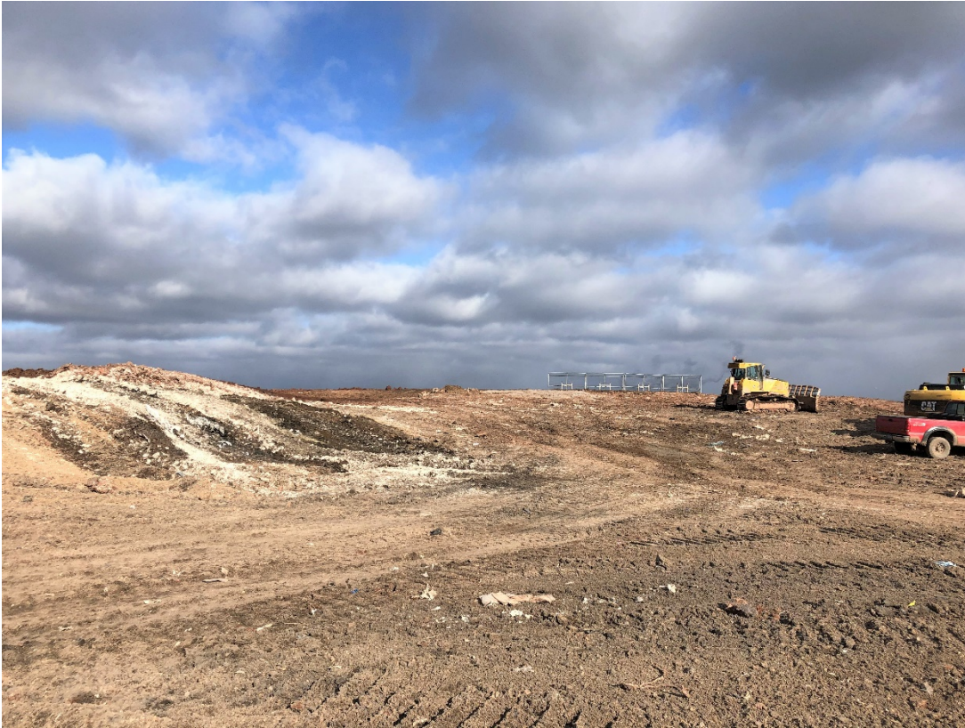
Photo 3: Location 2 – Looking North, Phase 3/4 Upper Lifts
