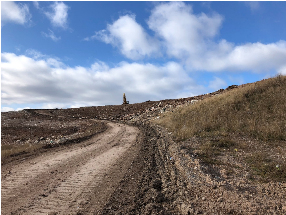
Photo 8: Location 5 – Looking Southwest, Phase 1 Southern Access Road
