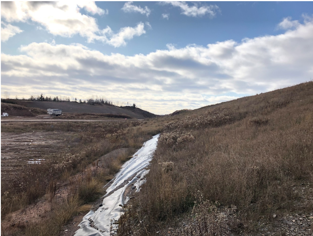
Photo 6: Location 4 – Looking South, Phase 1 Eastern Berm
