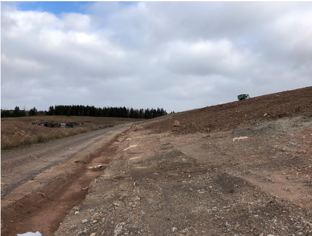
Photo 14: Location 8 – Looking North, Phase 3 Western Waste Slope
